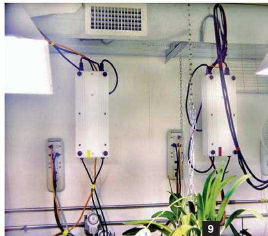
[9] Part of a wall in the warm room. The large white rectangular structures with electrical cables at each end are the ballasts for HID lights in that room. Each ballast box contains two ballasts — one for each 400 watt bulb in a reflector. Each reflector has a separate ballast box.
